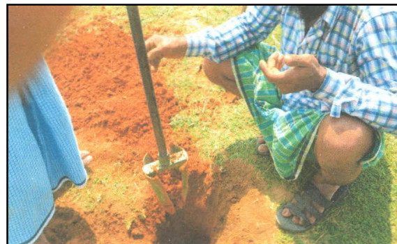
Figure 4.2: Extracting soil from bore-hole.
