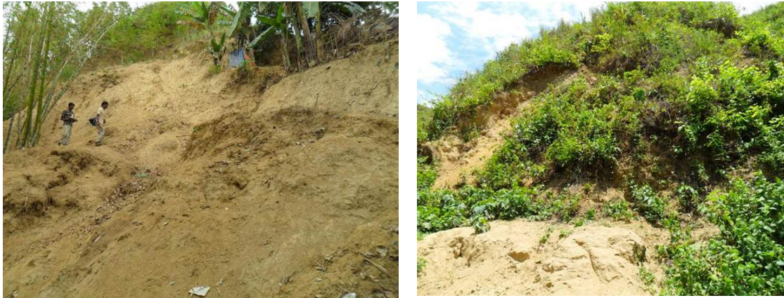
Landslide Sites at Puran Pallan Para
