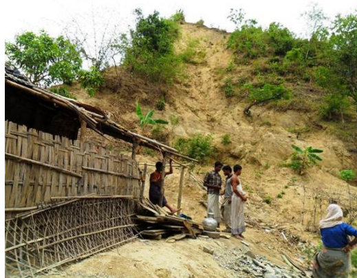
Houses Located near the Landslide site at Puran Pallan Para
