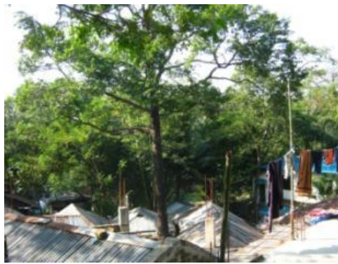
Houses vulnerable to Landslide-Mohajer para
