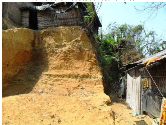
Vulnerable houses at Mohajer para
